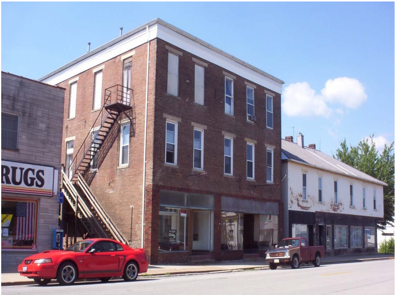
Downtown commercial area mixed uses and mixed-use buildings
